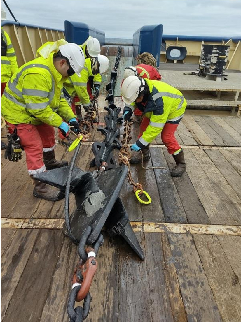
Cable recovered to deck by grapnel
